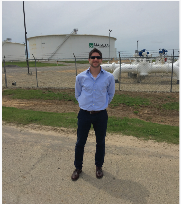
Magellan Midstream Partners’ crude oil tank farm in Cushing, OK. Magellan has the 3 rd largest storage capacity in the area with 14 million barrels in three different tank farm locations.
