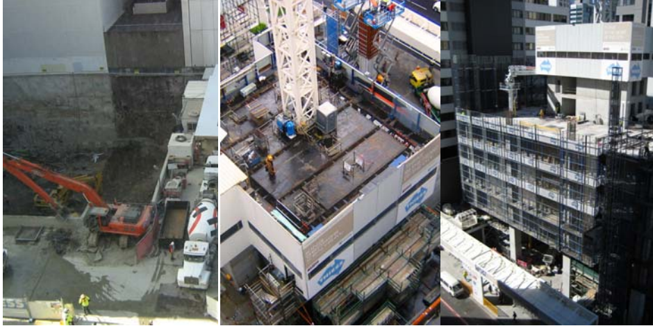
145 Ann Street, Brisbane (under construction)
