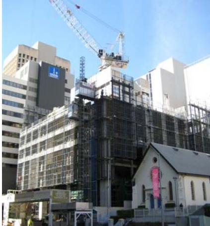
Construction works at 145 Ann Street, Brisbane
