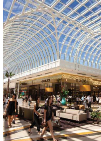
Chadstone Shopping Centre, VIC
