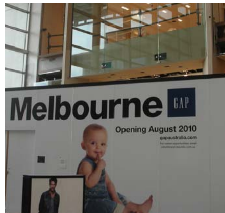
New GAP store being fitted out at Chadstone Shopping Centre, VIC
