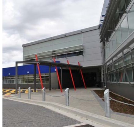
DHS Facility, Elizabeth Shopping Centre, SA
