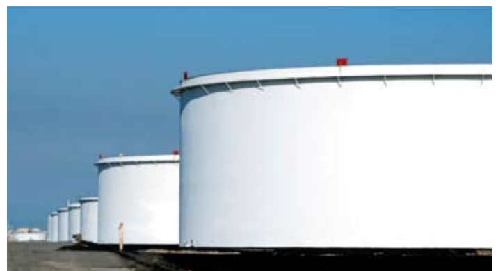
Energy infrastructure – oil storage tanks.
